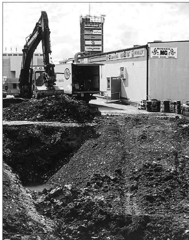
**Figure 2.2 Remediation of soil.** Old filling stations are sites where the soil is routinely monitored for chemicals before new uses. Here the soil under a previous gas station is being removed for a new residential house. (Photo: Lars Rydén)
