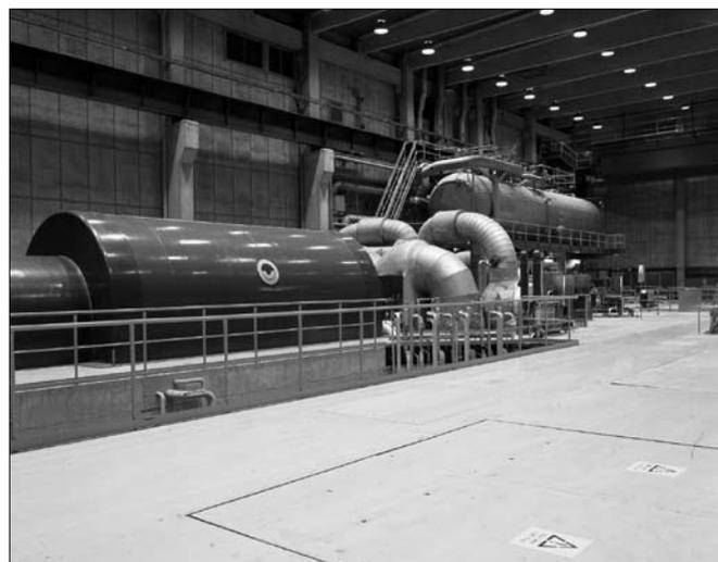
**Figure 6.5 Cogeneration.** Combustion for heat production may be coupled to electricity generation in turbines, as in this turbine hall. When the hot steam is pressed through the turbines electricity is generated. The steam is cooled to temperatures appropriate for the district heating system. With this combined system efficiency is close to the theoretical maximum. (Photo: Kjell-Arne Larsson)
