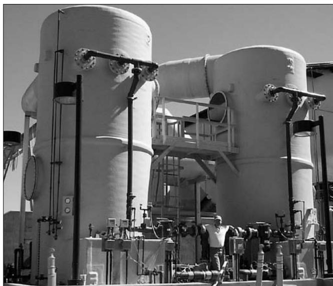
**Figure 9.7 Multi-stage packed chemical scrubbers.** These scrubbers are designed to remove hydrogen sulphide ( $H_2S$ ) based on neutralisation of the  $H_2S$  into a caustic solution. Recirculation increases the concentration of the gas in solution and decreases the quantity of scrubbing solution required. (Photo: www.bayprod.com)
